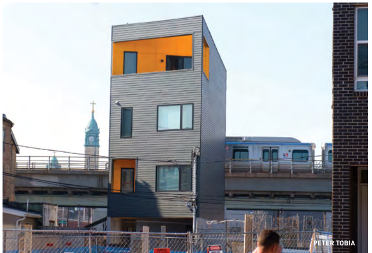
New housing construction in Point Breeze and along SEPTA’S Market Frankford line in Fishtown
