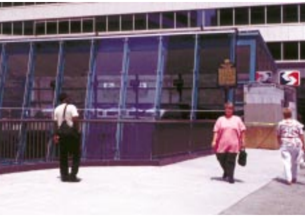
SEPTA's new glass-enclosed headhouse entrance at 15th and Market.
