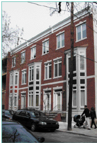
This newly constructed three-home infill development on 6th Street in Queen Village took advantage of the 10-year tax abatement for new construction. The 4,000-square foot row homes, marketed for $600,000, have been sold.
