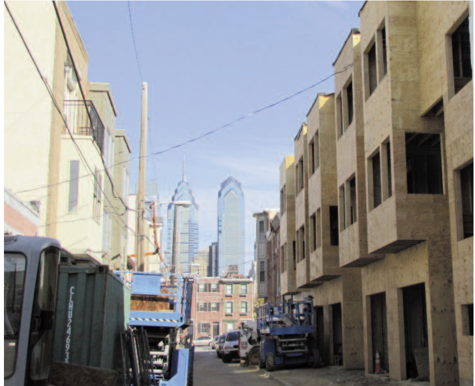
From South Philadelphia to Northern Liberties, infill and new construction has continued adjacent to downtown.
