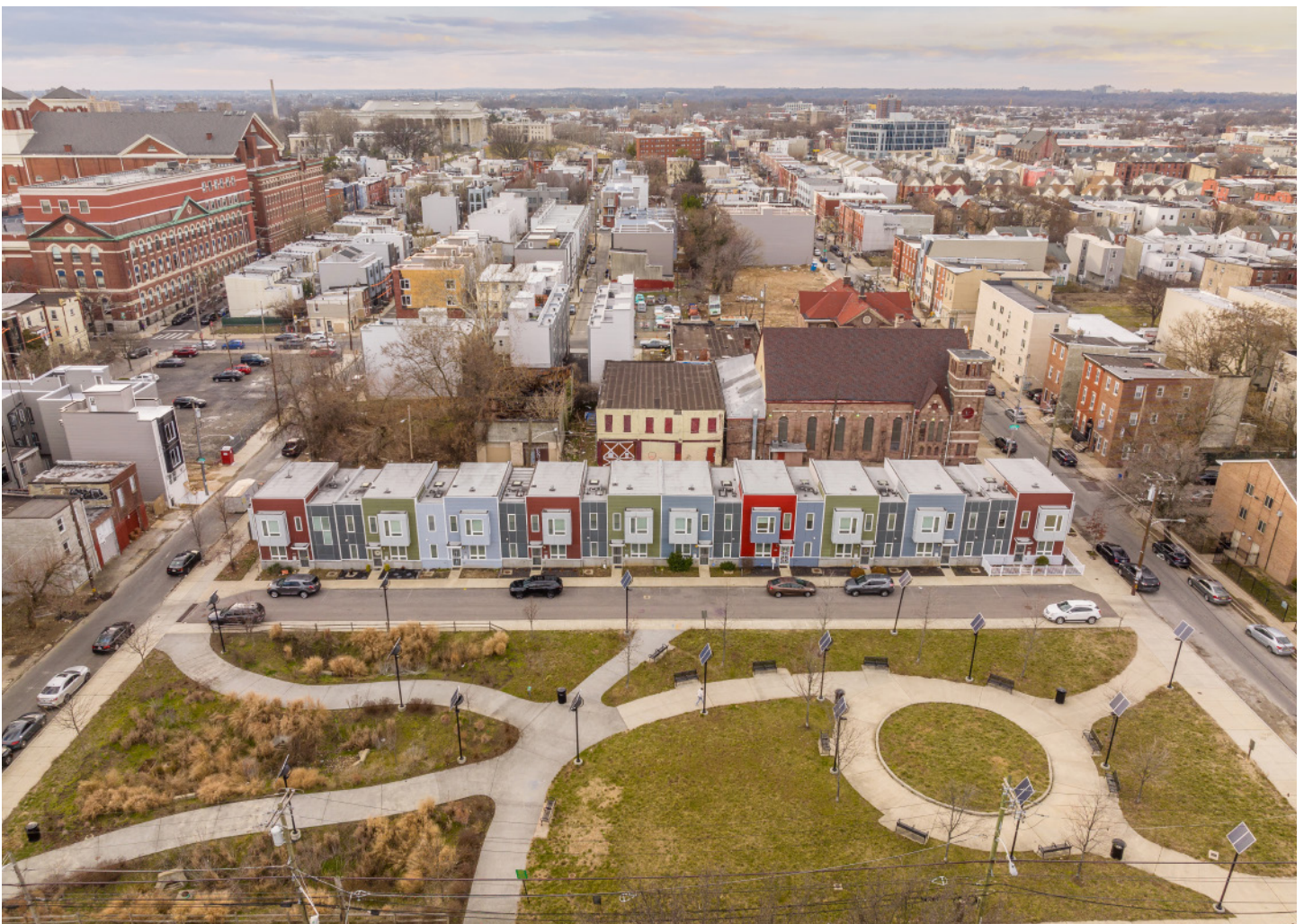
Located at North 16th and Market, the Ingersoll Commons, adjacent to Ingersoll Park, provides affordable housing adjacent to a new park with storm water mitigation features, the result of a partnership between Community Ventures, Philadelphia Water Department, and Philadelphia Parks and Recreation.
